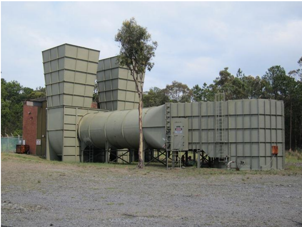
Plate 7.6: Mannering main ventilation fans
