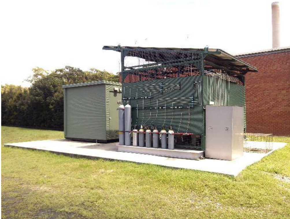
Plate 7.14: Chain Valley tube bundle monitoring (main winder and switchroom building behind)
