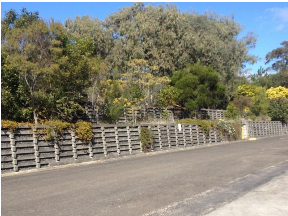
Plate 7.8: Mannering retaining wall below main carpark
